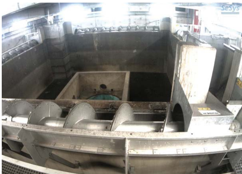
Typical camera image - pumps within a storm drain
